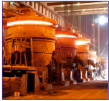
IRON & STEEL PLANT
